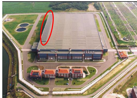
ZLN facility (red circle = storage hall 8)
