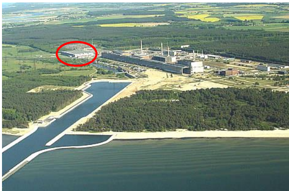
Premises of Energiewerke Nord GmbH at the Baltic Sea
