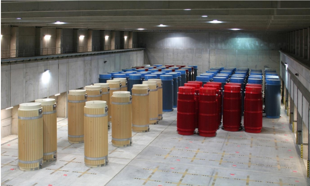
Figure 1: DPCs in an Interim Storage Facility Gorleben (Photo: GNS)
