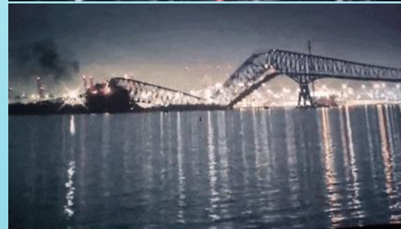
Baltimore Key Bridge, Maryland, US, March 26, 2024
