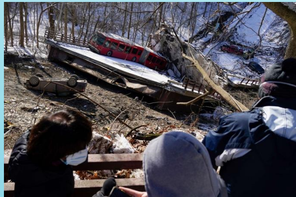
Human biased in bridge inspection
