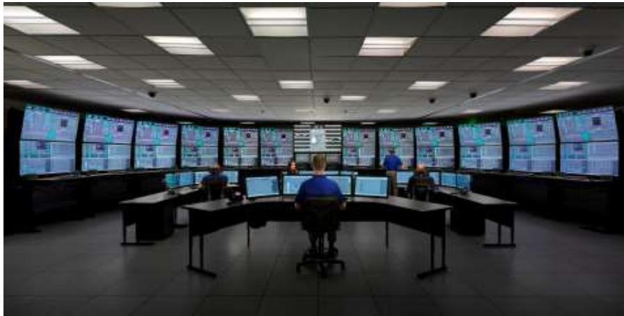
Figure 2: The NuScale concept main control room [9]
