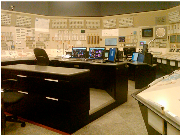
Figure 1. Example of a mostly analog I&C nuclear power plant main control room
