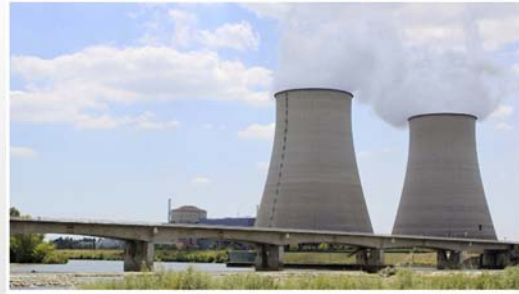
EPRI Assesses Seismic Resistance of Electronic Components
